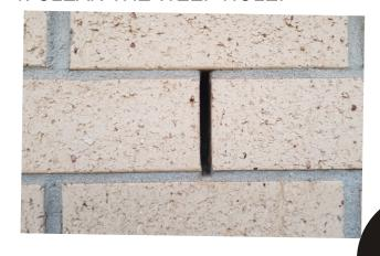
2. BY SQUEEZE THE CLIPS OF "WEEP HOLE COVER" SLIDE IT INTO WEEP CAVITY.
